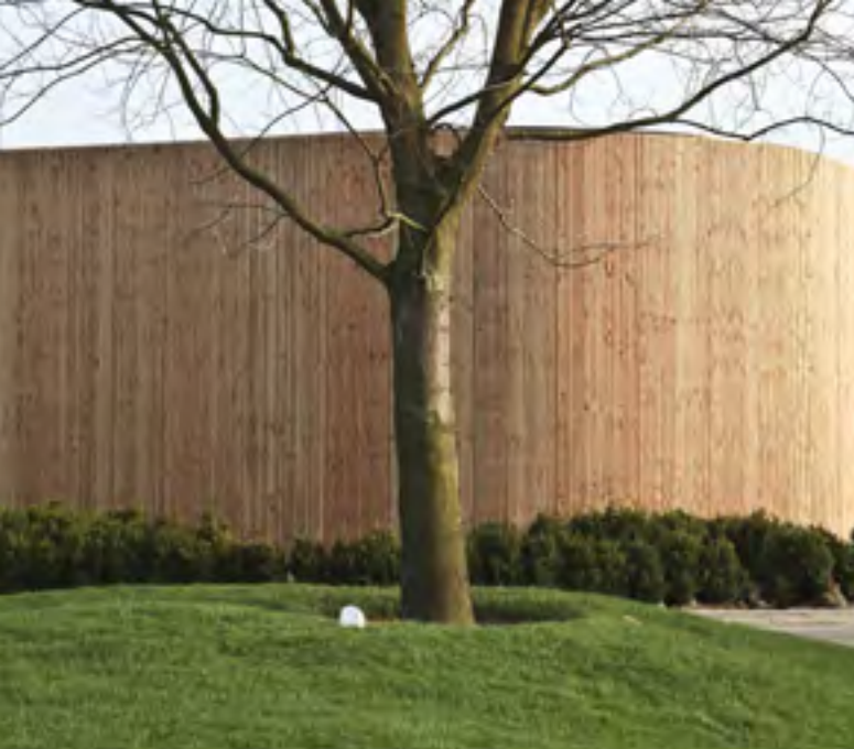
↑ Inground projectors in special steel tubes
