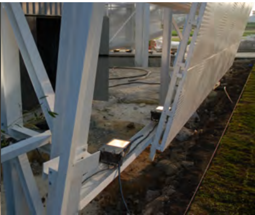
↑ Inground projectors in special steel tubes to protect from leaves ↓ Affordable fixtures in the inner-skin of the accesses.
