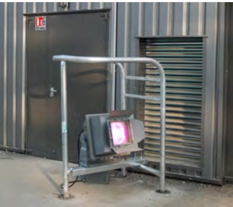
↑ Underline of the main paths with projectors placed on parking poles. ↓ Color changer fixtures in the inner-skin, protected by steel tubes
